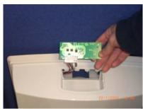
Remove control panel and replace with new
