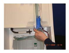
Replace the fuse and holding tank, add a couple of litres of water to the flush tank and test.
