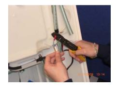
G Reconnect the flush tube to the top of the pump
